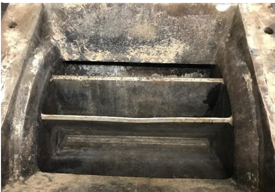
View of the rotor (note bent blade)
